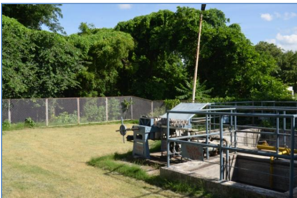
Sewage Treatment Plant
