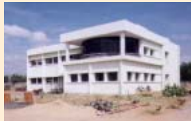
Nuclear Desalination Demonstration Plant (Capacity : 6300 cubic metre per day) set up at Kalpakkam, Tamil Nadu
