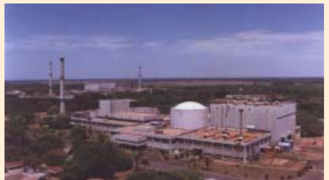
Fast Breeder Test Reactor at IGCAR, Kalpakkam, Tamil Nadu
