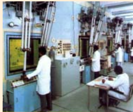
Radioisotope production facility at BARC
